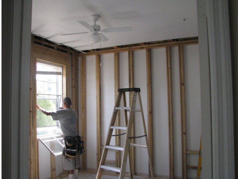
Photo #3 – Installation of interior shoring walls at Building 24.
