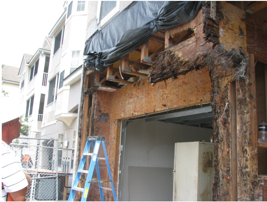
Photo #2 – Rot decayed wall framing at Building 41.
