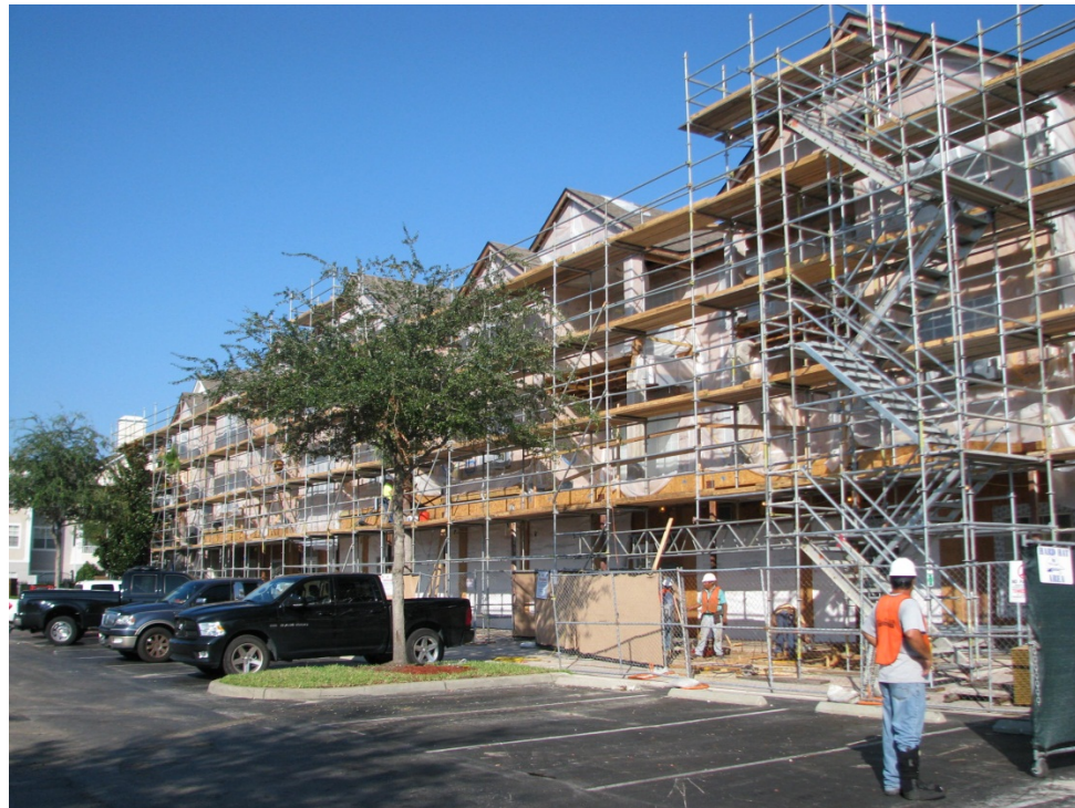
Photo #5 – Repair scaffolding.
